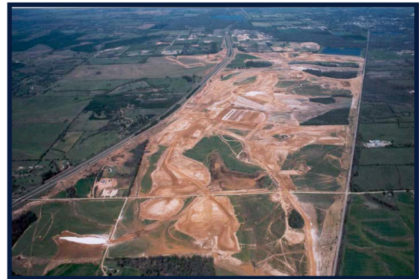
Construction of Building Pad March 2001
