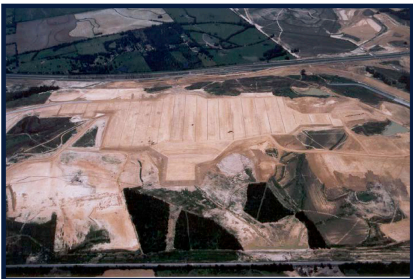
Completed Building Pad April 2001
