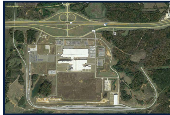
Toyota Manufacturing Plant Today
