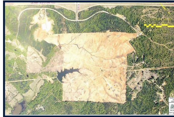
Completion of Clearing & Grubbing Building Pad April 2007
